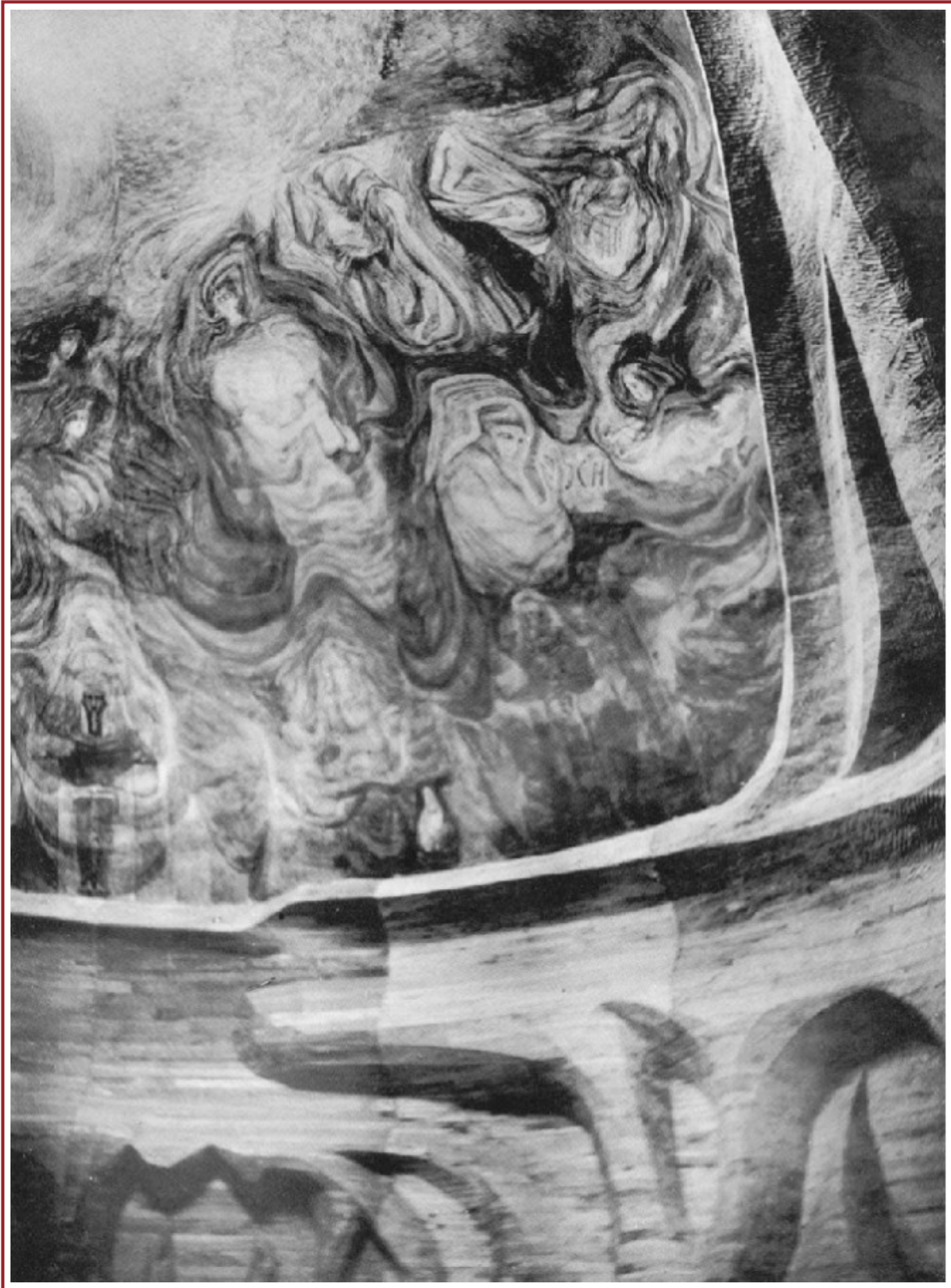
Interior of the Roof. Section of the architrave motif and frescoes in the small Cupola
