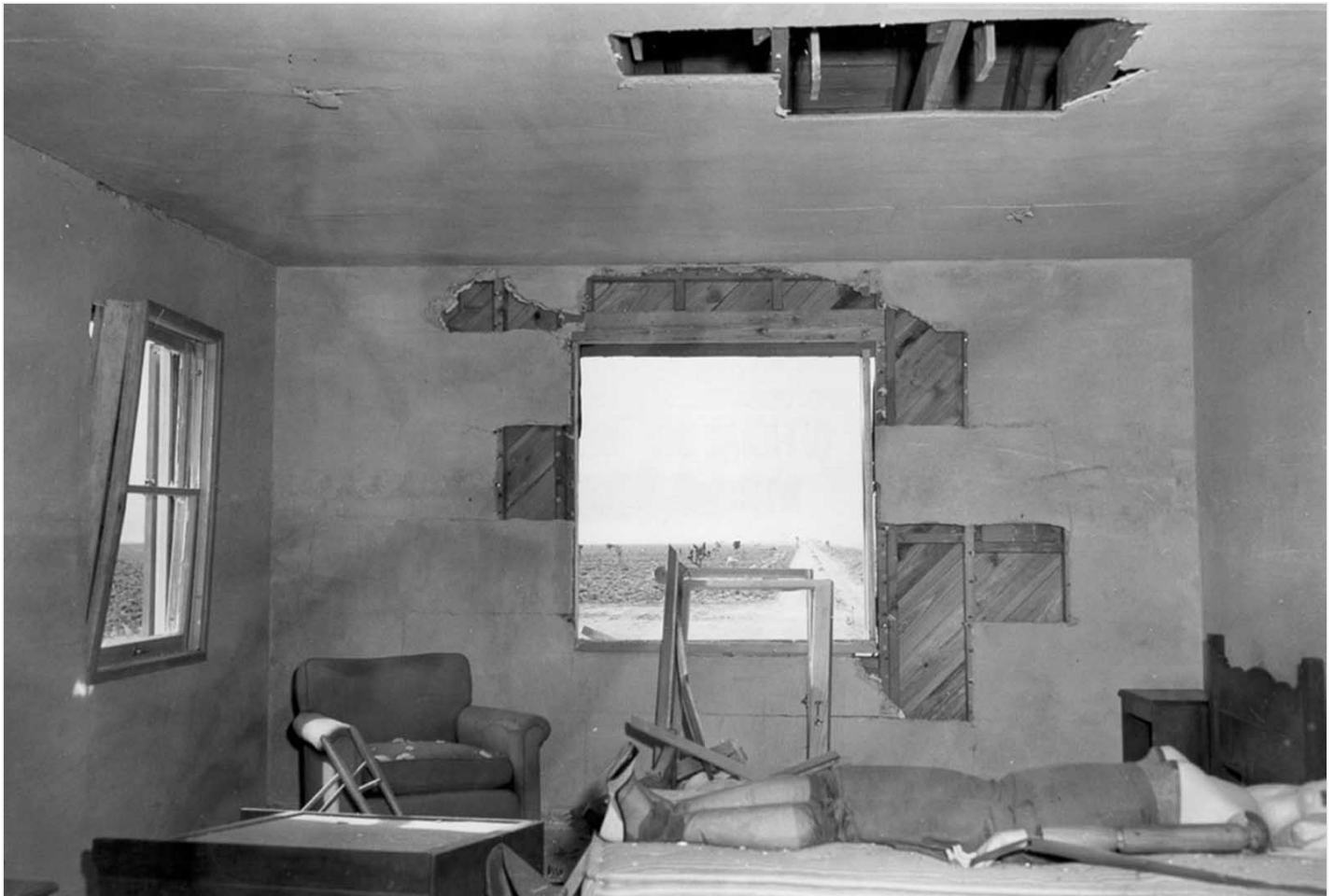
(2 of 2) After the blast, a damaged bedroom, window, and blankets missing, resulting from a test during an atomic blast on March 17, 1953.
