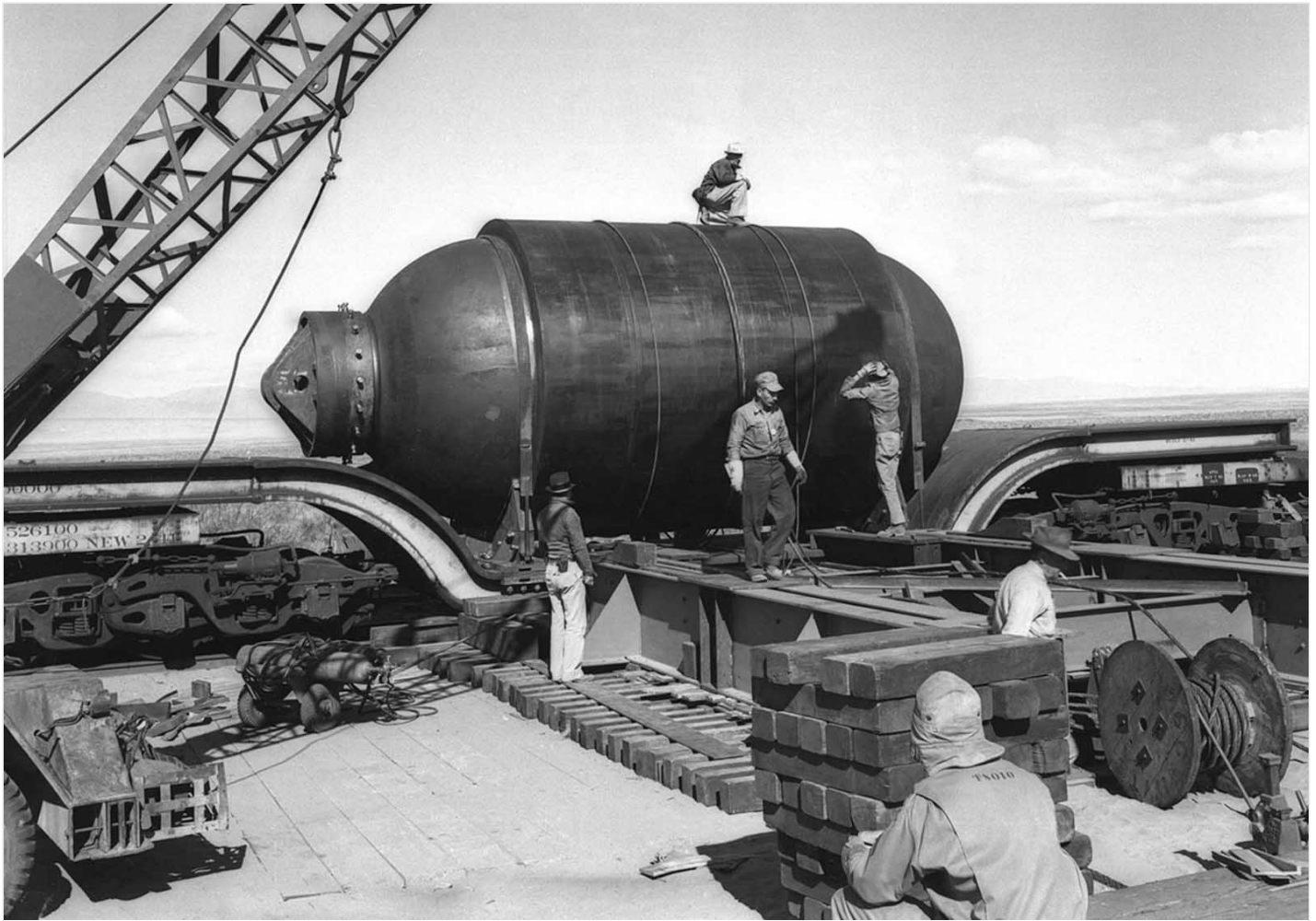
Jumbo, a 200-ton steel canister designed to recover the plutonium used in the Trinity test in the event that the explosives used were unable to trigger a chain reaction. In the end, Jumbo wasn't used for recovery but was placed near ground zero to help gauge the effects of the blast. It survived intact, but its support tower did not.
