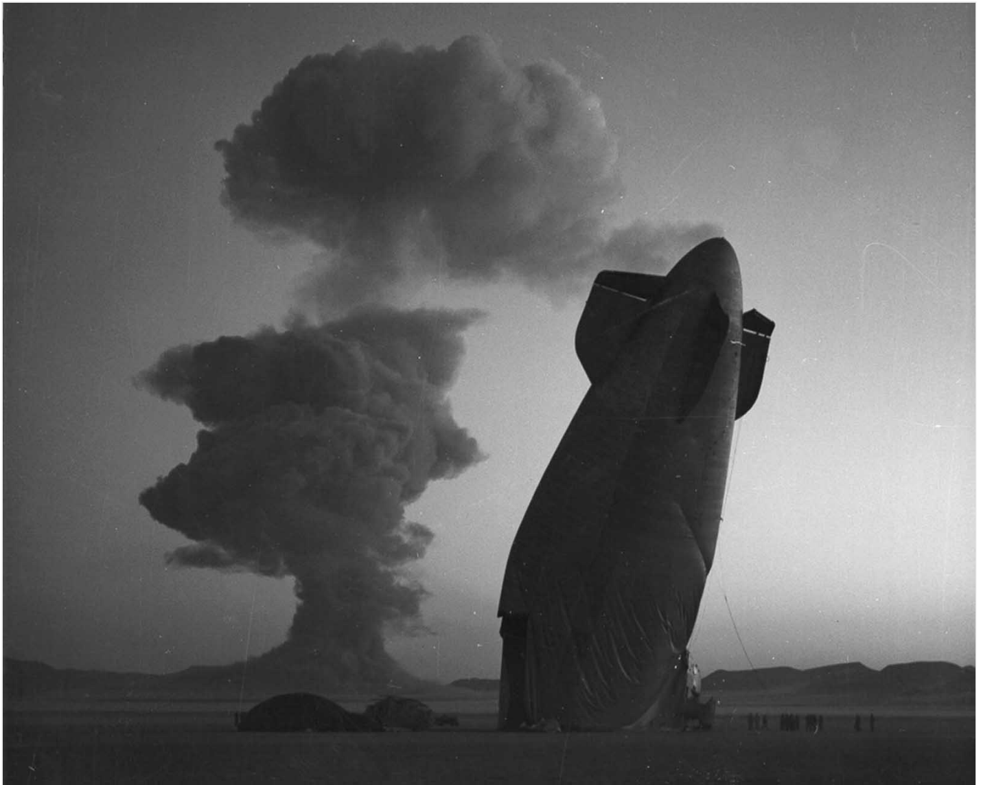
The tail section of a U.S. Navy blimp is shown with the Stokes cloud in the background at the Nevada Test Site on August 7, 1957. The blimp was in temporary free flight in excess of five miles from ground zero when it was collapsed by the shock wave from the blast. The airship was unmanned and was used in a military effects experiment.
