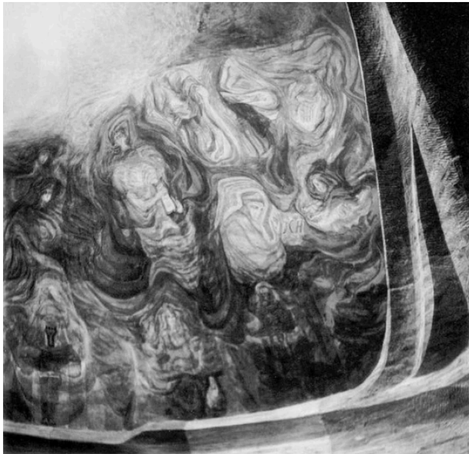
71. East cupola, southwest side
