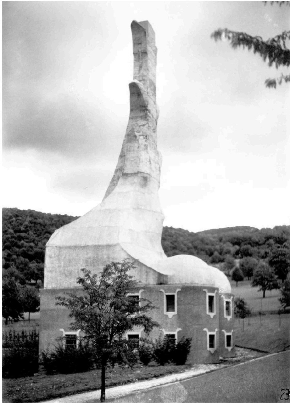
100. Heating house from the southwest
